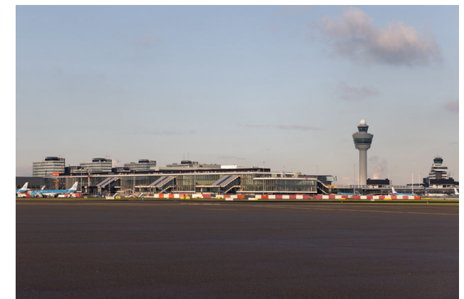
The new Pier A is necessary to guarantee the future demand for new aircraft stands and gates, but also to create redundant capacity to be able to renew or refurbish existing piers.
